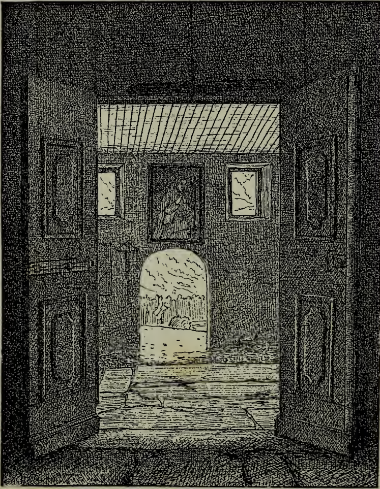
ROSSURA CHURCH PORCH IN 1879.
